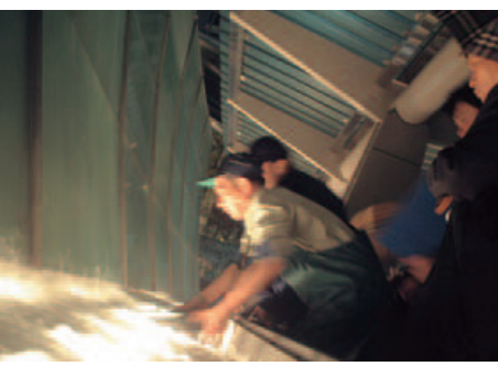
28. 66プラザの水景施設の光が未調整である。水中照明の位置や照射角度を指示。 28. Giving instructions on the positions and angles of lights for the aquascape of the 66 Plaza, the lighting for which had yet to be adjusted.
